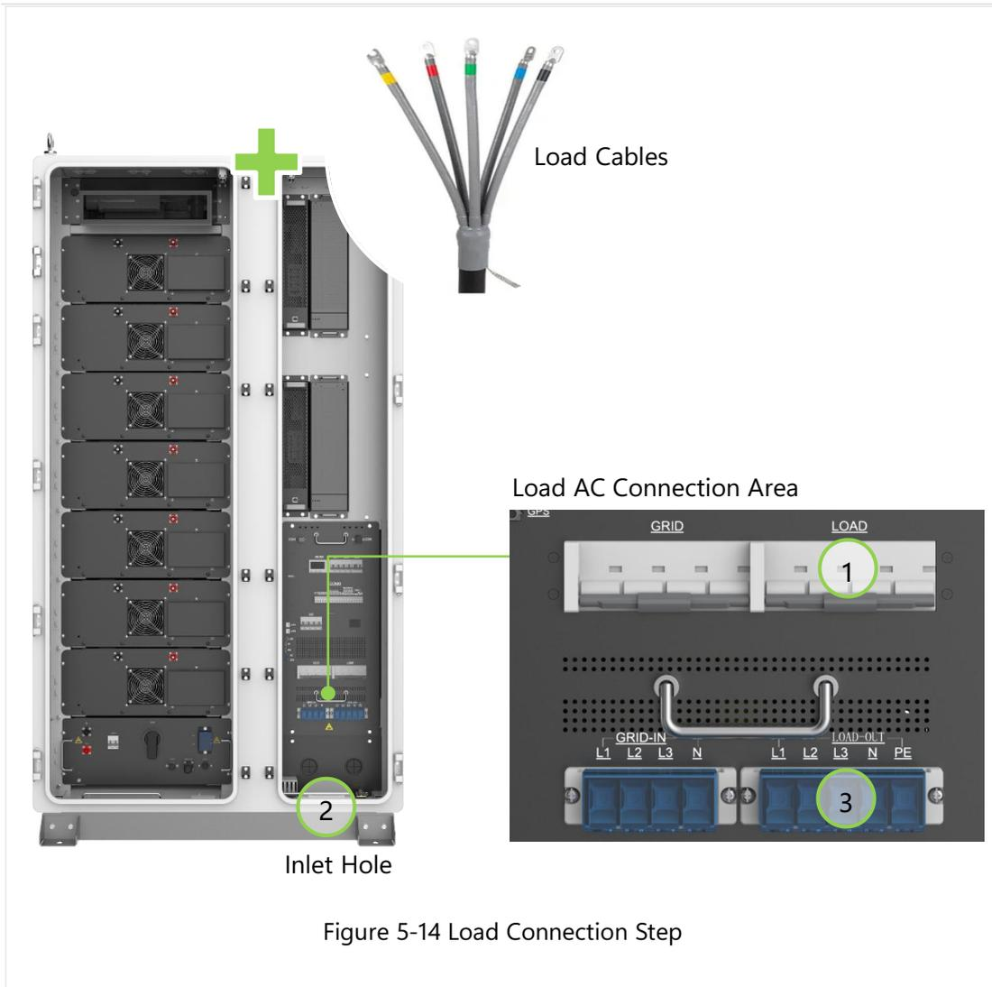
Figure 5-14 Load Connection Step
